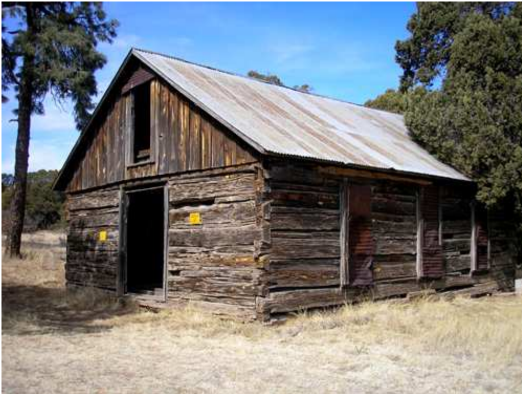
Figure 5 Log Schoolhouse in Jicarilla, New Mexico (Photo by author, 2016)
