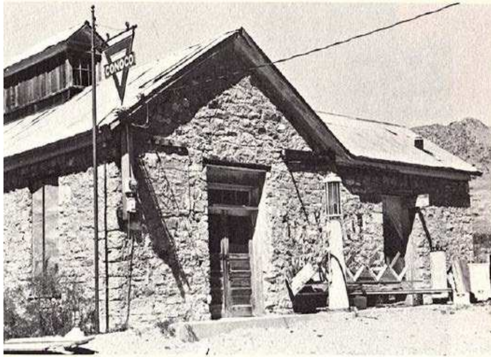
Figure 24 1893 Schoolhouse showing reuse as a gas station. Note the Addition of the Ventilation Cupola on the center of the roof. Phot originally published in Ghost Towns and Mining Camps of New Mexico , by James E. Sherman and Barbara H. Sherman. Copyright © 1975 University of Oklahoma Press. Reprinted by permission of the publisher.
